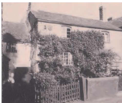
Clifton Cottage, Mill Street
