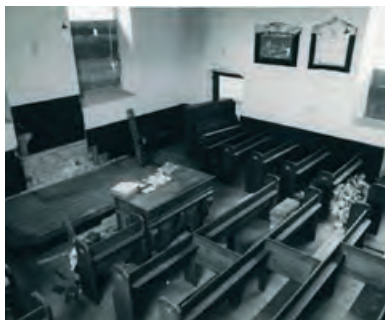
A view of the interior at the time of purchase
