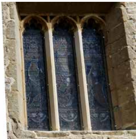
After, new mullions, releading & new guards
